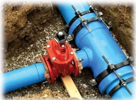
New PVC watermain to replace old ductile iron watermain
